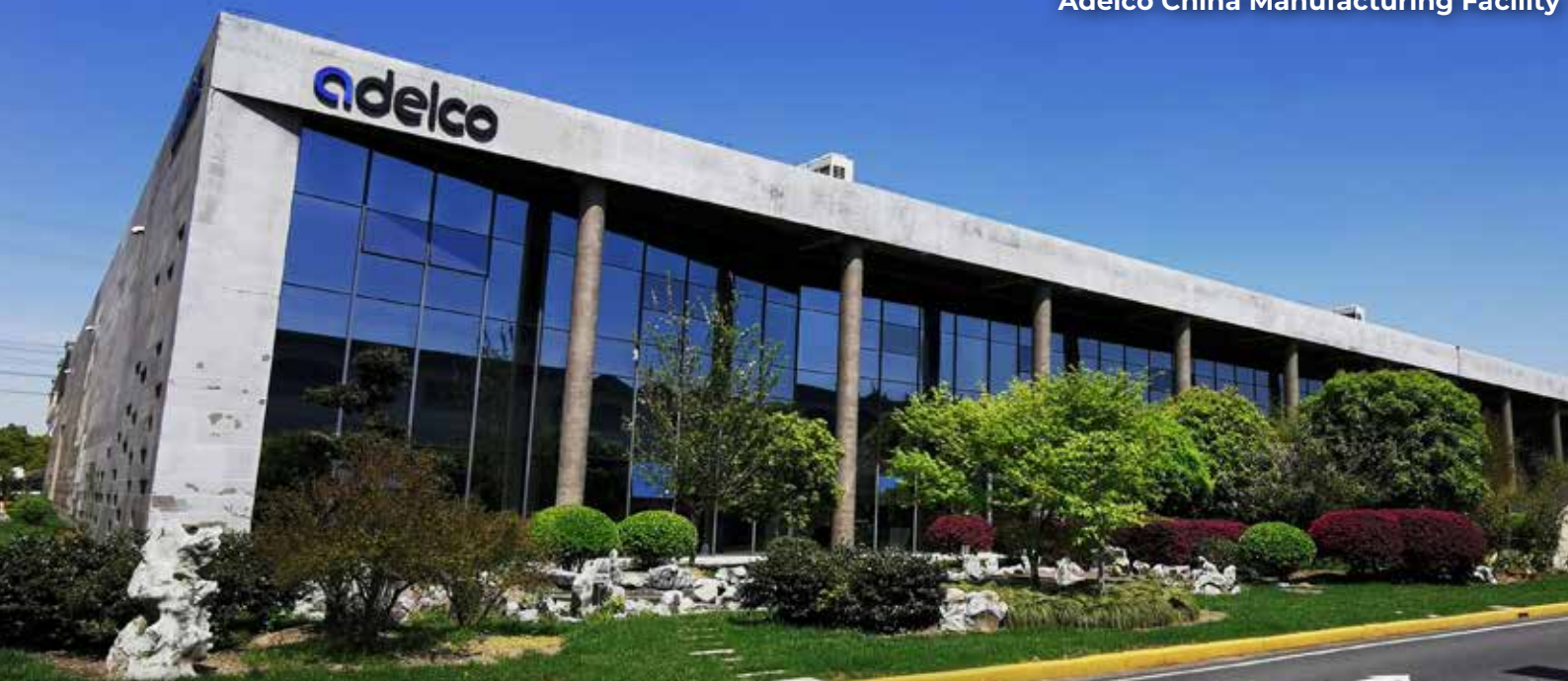
Adelco China Loading and Shipping Area
